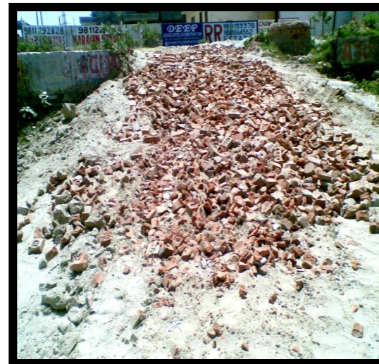
Gravel Road Entrance for Soil Erosion
