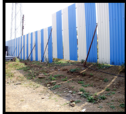
Sample picture of Barricading the Site Boundary
